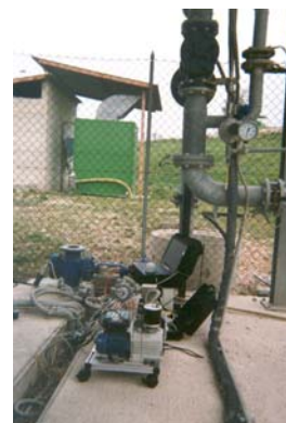
Figure 10 Landfill Site in Italy
